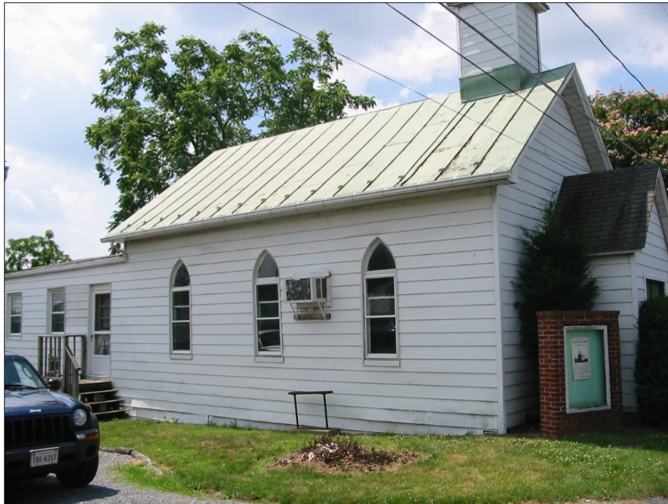
Figure 7. View of northeast elevation, showing standing-seam metal roof and lancet windows (History Matters, 2005).
