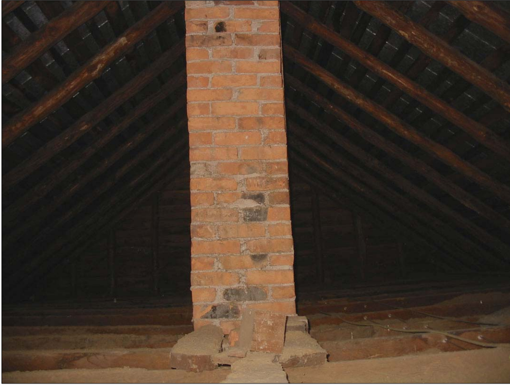
Figure 5. View of chimney in attic (History Matters, 2005).
